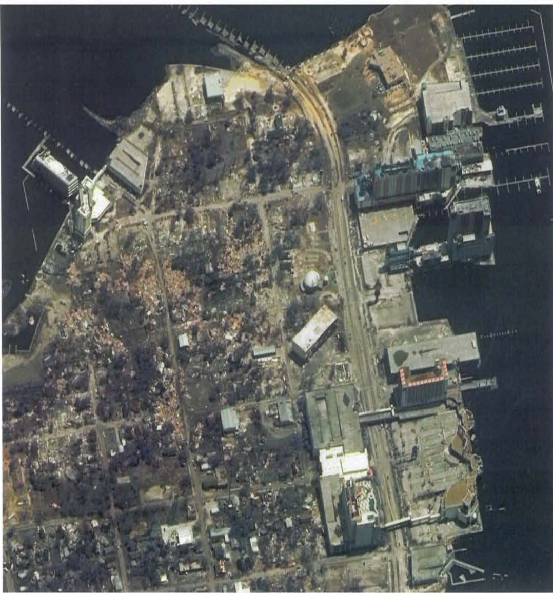
« Waterfront in Biloxi, Miss. following Hurricane Katrina, one of the most devastating storms in the U.S. in decades (Courtesy of Digital Globe).
